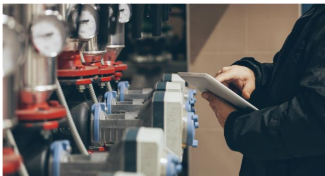
Motors and Drives System Audit
